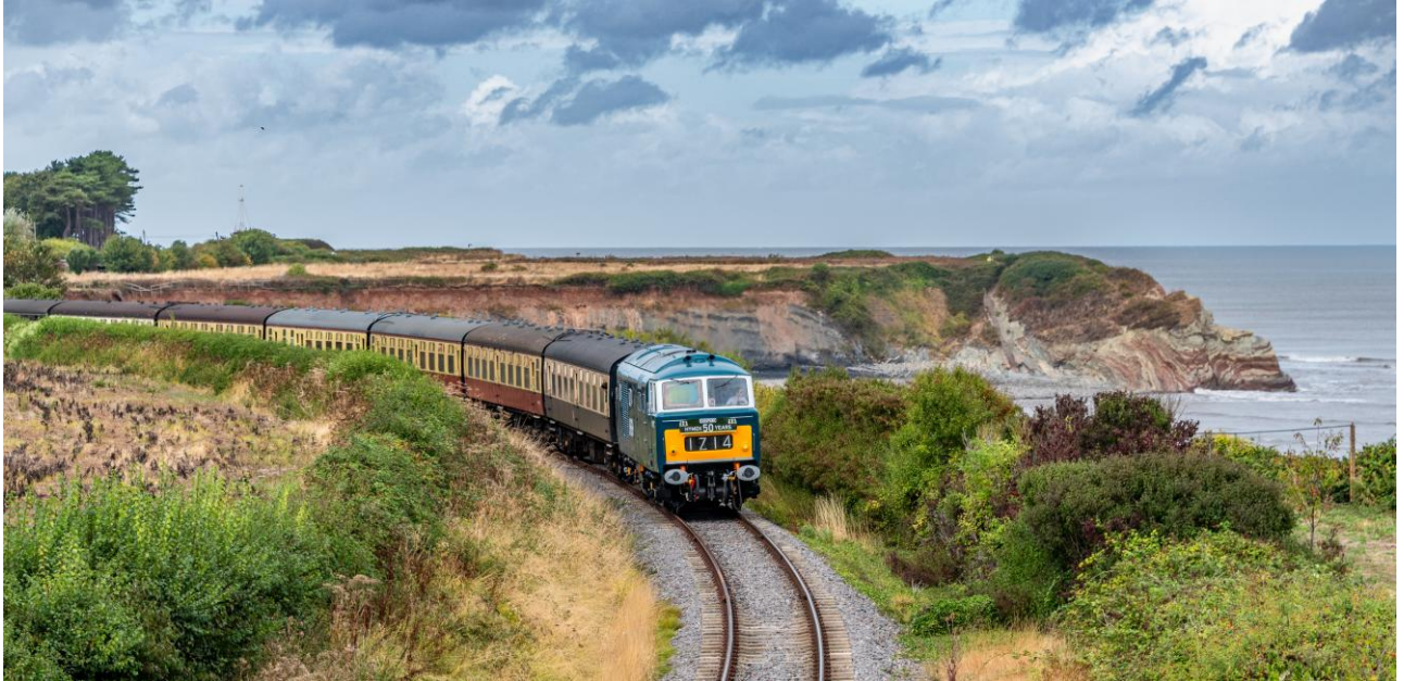
DEPG Hymek D7017 approaching Doniford Station. One of the challenges facing the Railway is coastal erosion at Helwell Bay along this stretch of the line.
